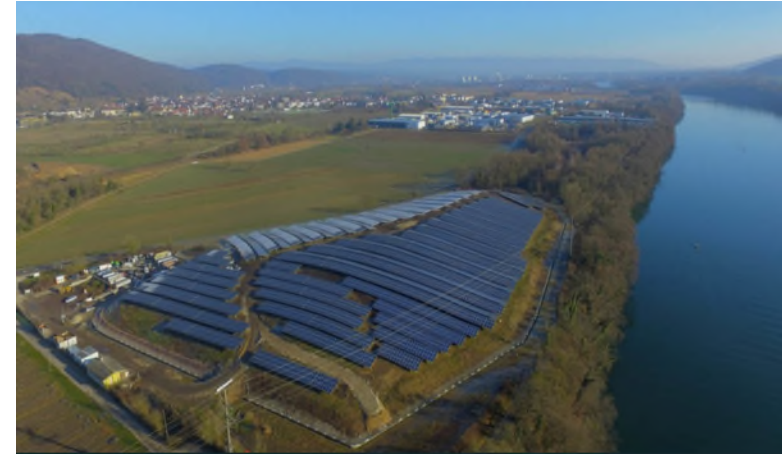
Solar Park at Herten - EWS Schönau, Germany
